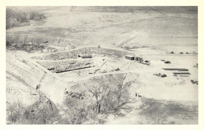
An aerial view of the diversion dam being built on Wet Walnut creek. The diamond-shaped earthern structure surrounds the site for the dam and blocks off Wet Walnut creek, which can be seen skirting the lower left-hand corner of the earthworks via a diversion ditch. Photos courtesy of Great Bend Tribune.
