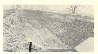
A mile west of where the diversion canal enters the Bottoms, a "drop-structure" has been built. This device, whereby the water drops twenty feet, will slow down erosion and scouring. The water falls into a "stilling basin," or "energy dissipator," that permits it to flow on into the Bottoms at a leisurely pace. The above picture shows the downstream side of the drop structure.
